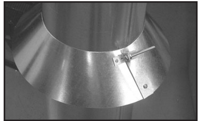
Figure 7.11 insert Bolt into Brackets
