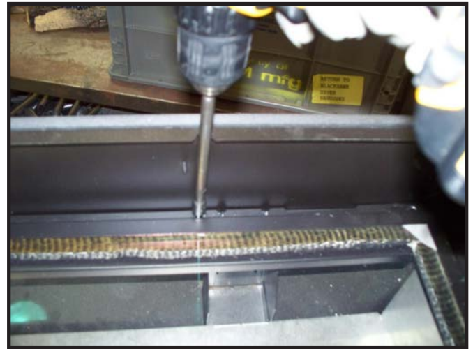
Figure 9.4. Gas and Electrical Access - Remove Glass Window
