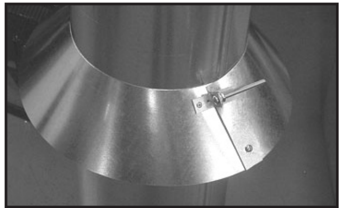
Figure 7.10 insert Bolt into Brackets
