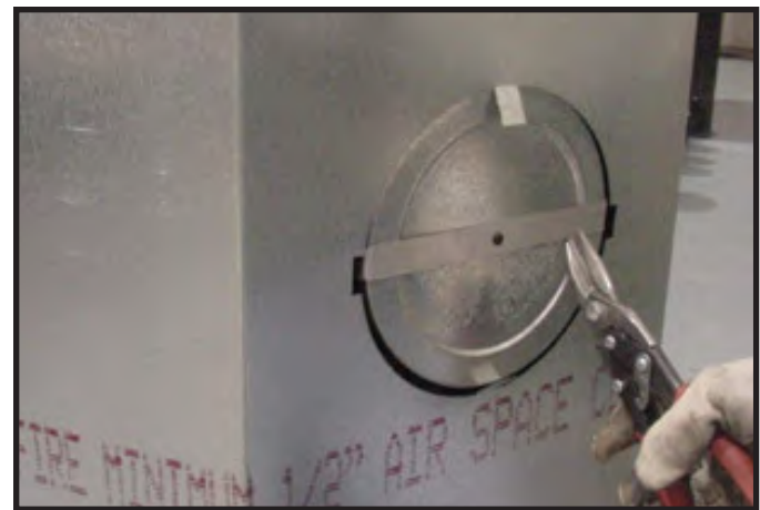
Figure 6.10 Cut the metal retaining band and fold the sides out.
