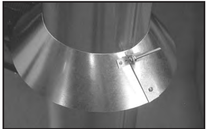
Figure 7.13 insert Bolt into Brackets
