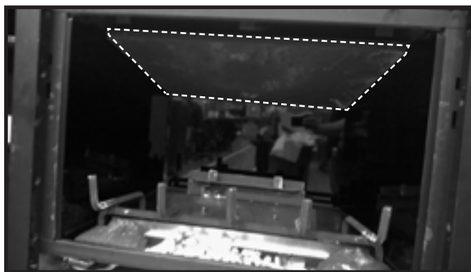
Figure 11.5 Install Top Refractory Panel
