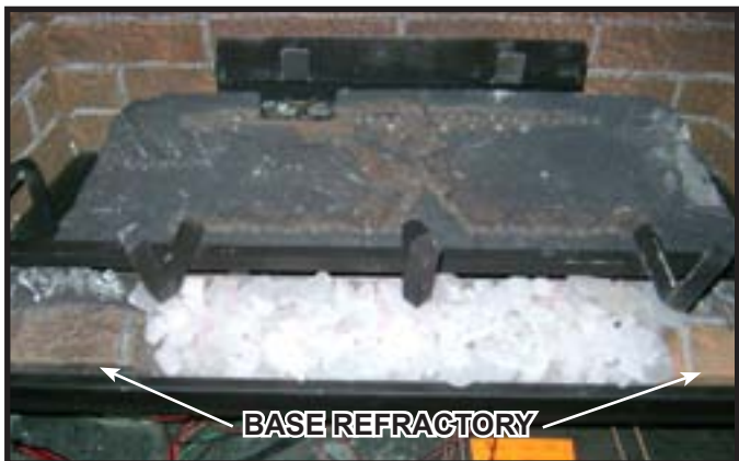
Figure 11.6 Install Base Refractory
