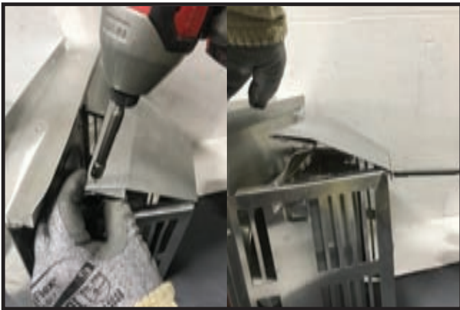
Figure 7.15 Wind Diverter Installed
