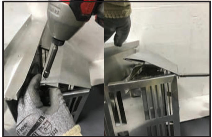
Figure 7.18 Wind Diverter Installed
