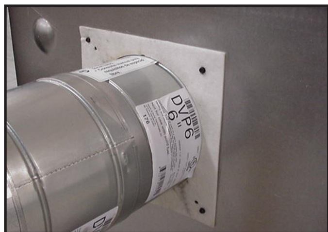
Figure 6.12 (Generic Appliance Shown) Attach the first vent section (it will snap into place). Slide the insulation gasket onto the vent section, up against the appliance and over the tabs. Use two self-tapping screws to secure gasket to outer wrap.
