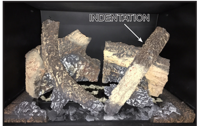
Figure 9. Top Right Log Installed - Log Set Complete
